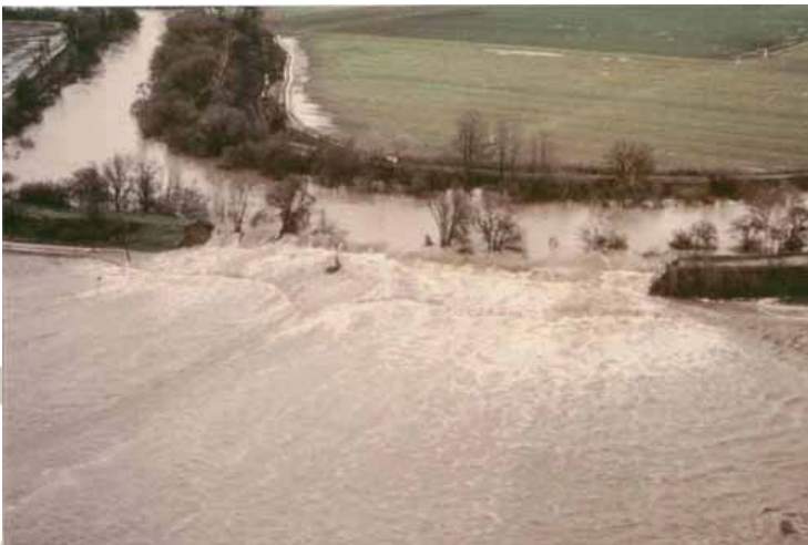
Figure 1.4: North-Eastern Levee Break at MWT
