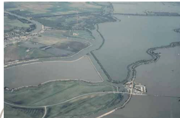
Figure 1.5: MWT Completely Inundated
