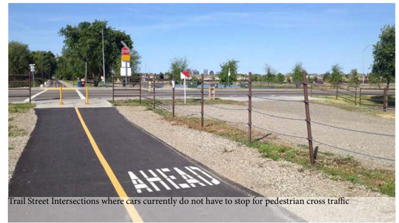
Signage along Clarksburg Branch Line Trail
