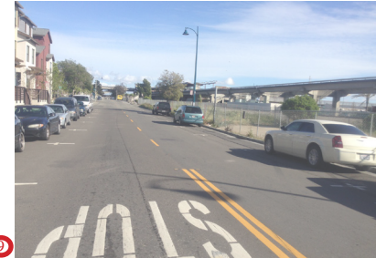
9 No sidewalk next to empty lot
