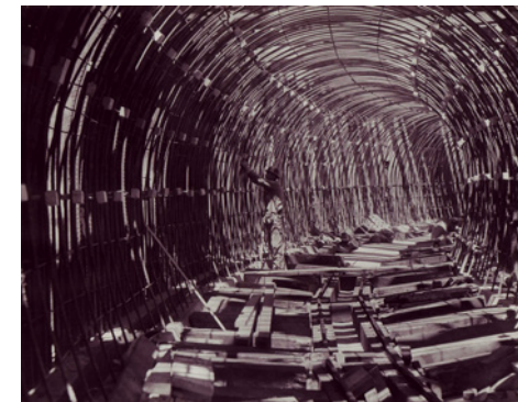
Fig 1.3: Construction of the LA sewer system
