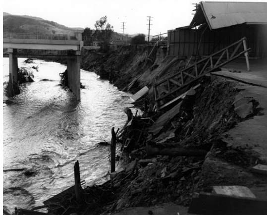
Fig 1.6: Bank Erosion during Flood of 1934
