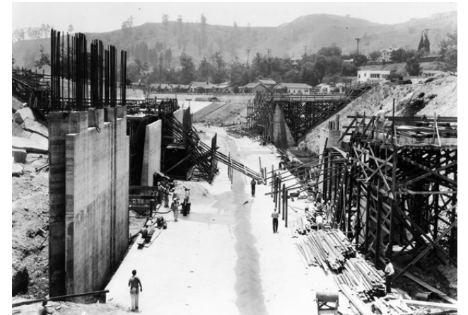
Fig 1.7: Channel Construction of the Arroyo Seco 1935
