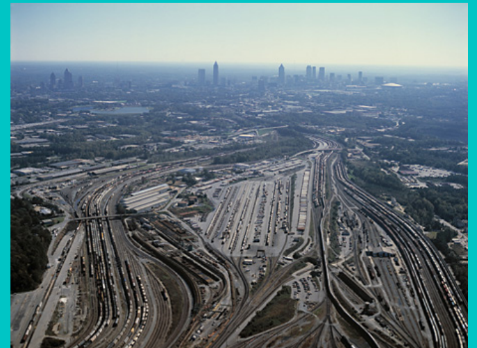
21 Rail Hub . Norfolk & CSX's Tilford Yard, Atlanta, Georgia
