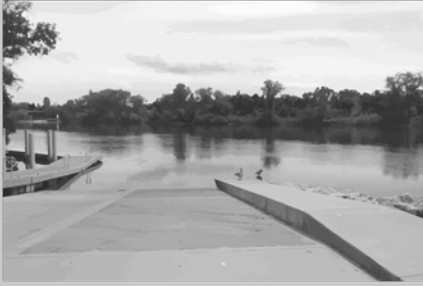
Typical boat ramp access point: concrete ramp with public restroom
