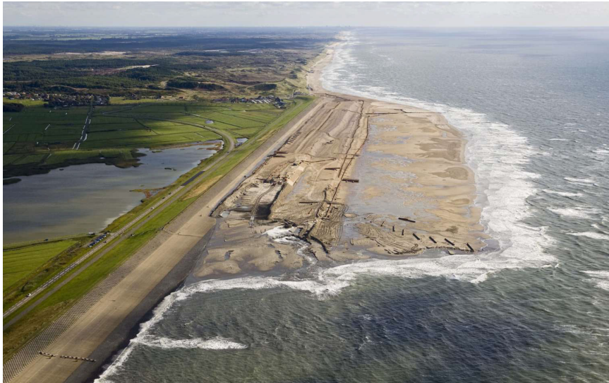
FIGURE 4-5 Construction of the Hondsbosse and Pettemer Sea Defense (Boskalis, 2015)
