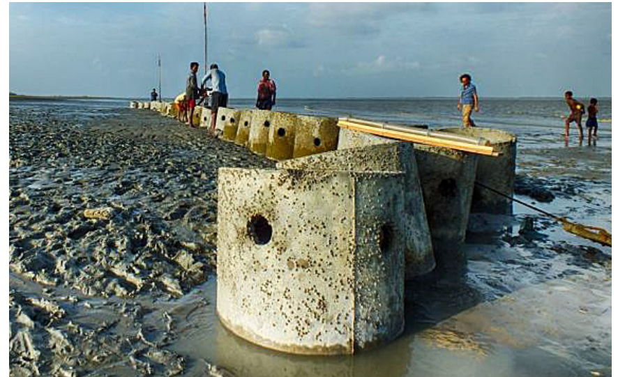
FIGURE 2-5 Artificial oyster reefs can prevent coastal erosion and grow fast in height to keep pace with sea level rise. (Netherlands Water Partnership, 2015)
