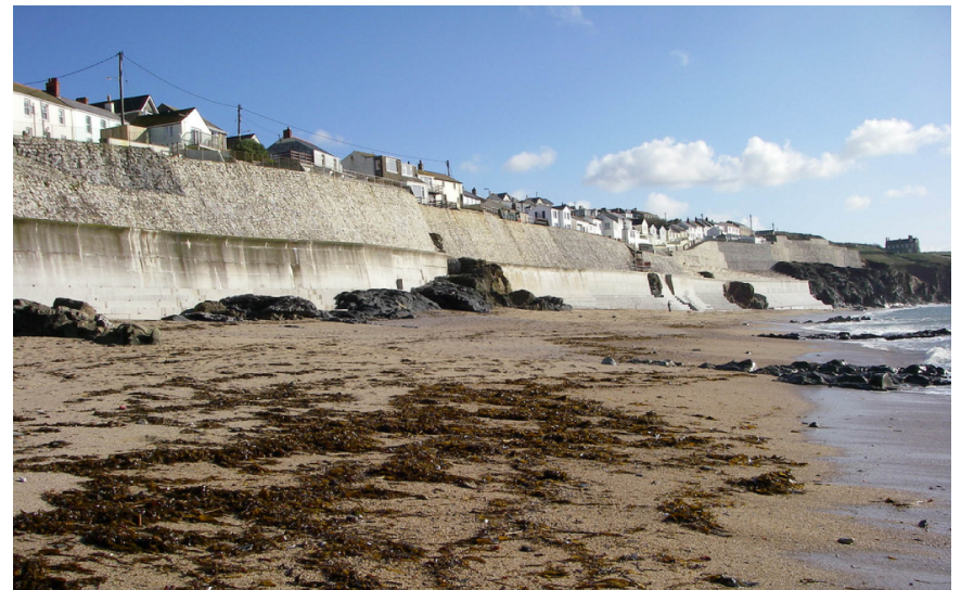
FIGURE 1-2 Massive concrete seawall along the coast and reduced beach space due to erosion (Granite, 2009)
