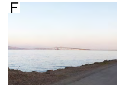
Fig. 4 - 7 Bridge ocean view
