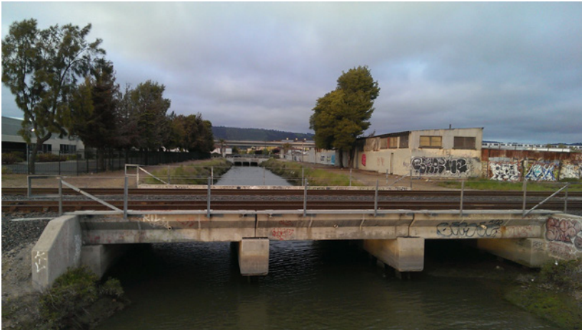
Figure 4.11 Railroad over the Lion Creek
