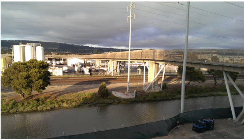
Figure 4.8 Skywalk over the slough
