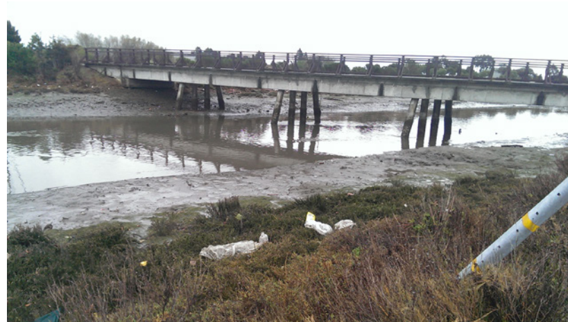
Figure 4.7 Pedestrian Bridge near the mouth of Damon Slough
