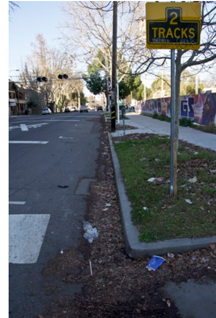
Figure 23 - 25 These images are the current conditions of 16th Street. It is hard to identify where the drains are located because they are covered with sediment. The stormwater facilities with help with the amount of sediment but there still will need to be some maintenance to clear curb cuts.
