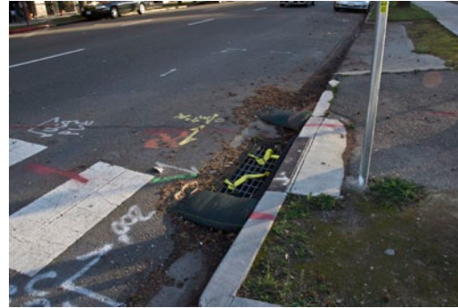
Figure 23 - 25 These images are the current conditions of 16th Street. It is hard to identify where the drains are located because they are covered with sediment. The stormwater facilities with help with the amount of sediment but there still will need to be some maintenance to clear curb cuts.
