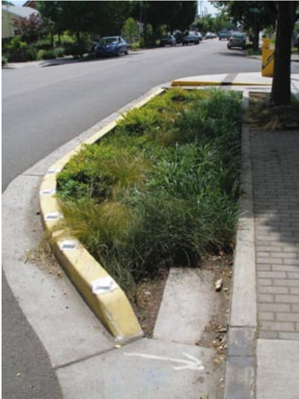
Figure 27 Curb cut in a curb extension. To make it most effective there needs to be a drop in grade to keep the water in the facility. 6" is the typical amount of grade change needed
