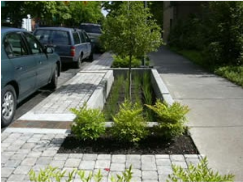
Figure 8-10 SW 12th Avenue and Montgomery St. in Portland, Oregon. Stormwater planters with pedestrian egress zone.
