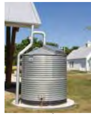
5.4 Cistern for storing rainwater runoff from the roof
