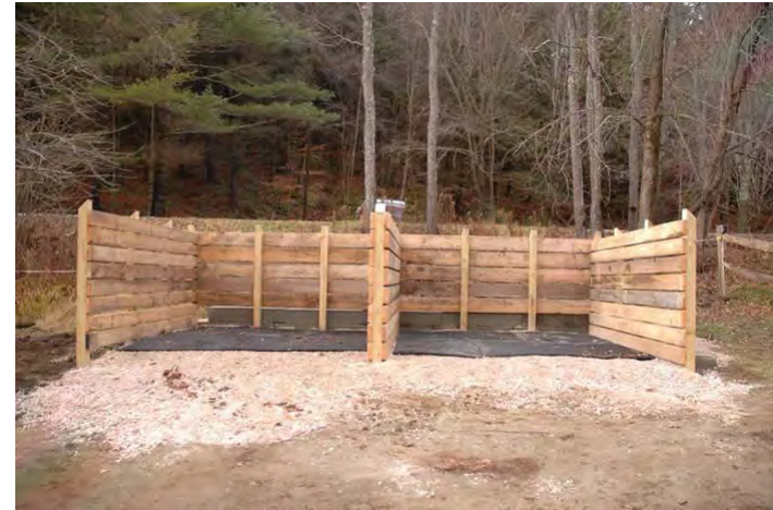
5.1 An example of compost bins
