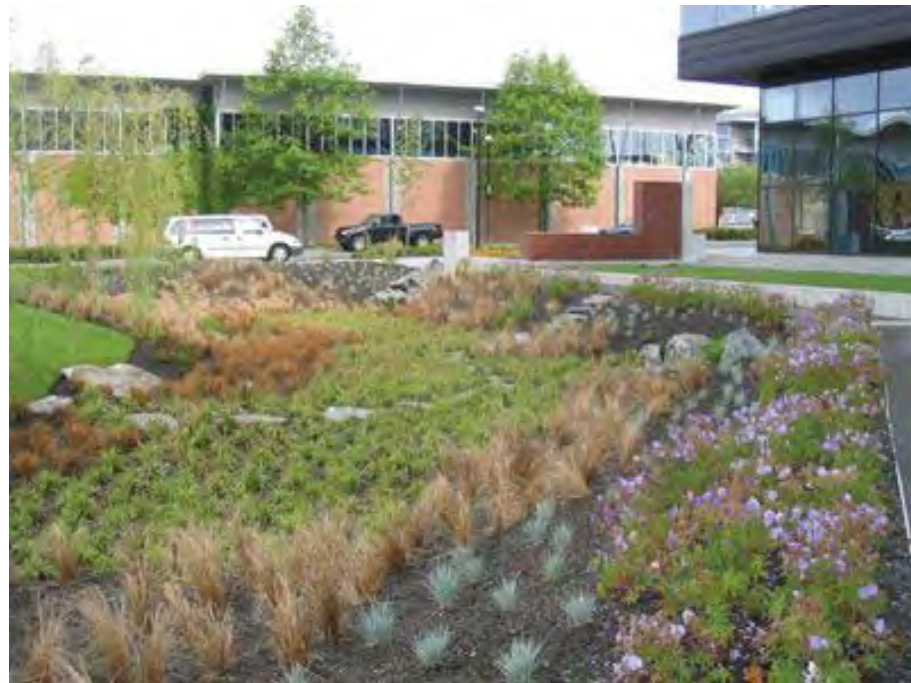
5.5 An example of a bio-swale with a variety of grasses
