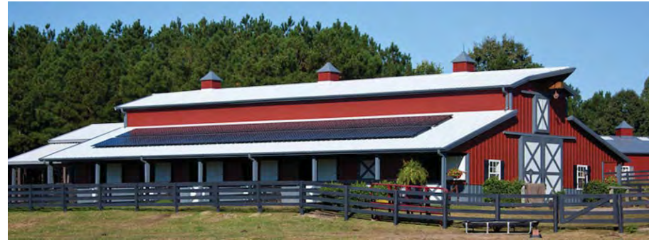
5.2 Photovoltaic panels on the roof of a barn
