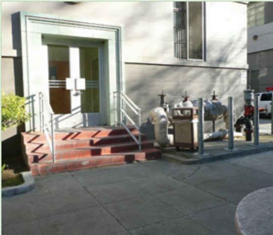
Figure 3.10 12th st. Entry 3 & Utility Pad
