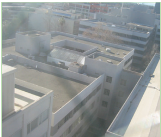
Fig. 3.13 South Building Roof & Alley
