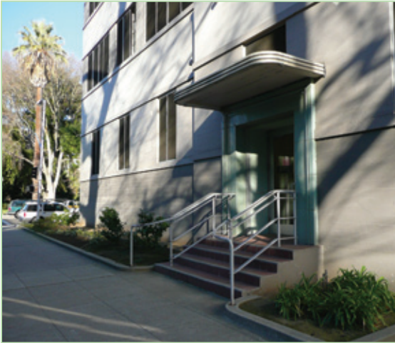
Figure 3.8 12th st. Entry 1 (West)
