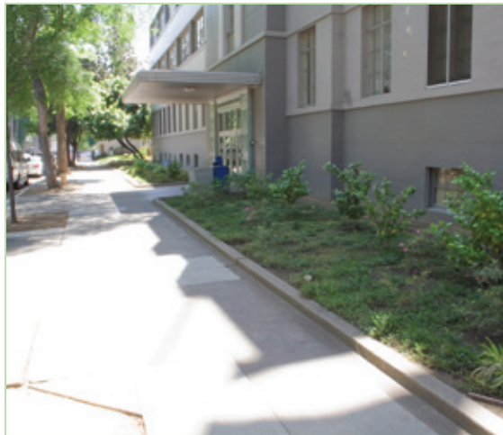
Figure 3.5 N st. Sidewalk Looking East
