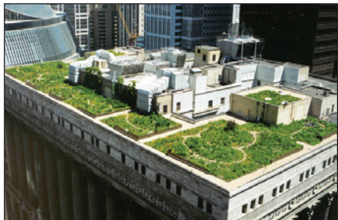
Figure 4.9 City of Chicago City Hall's Green Roof
