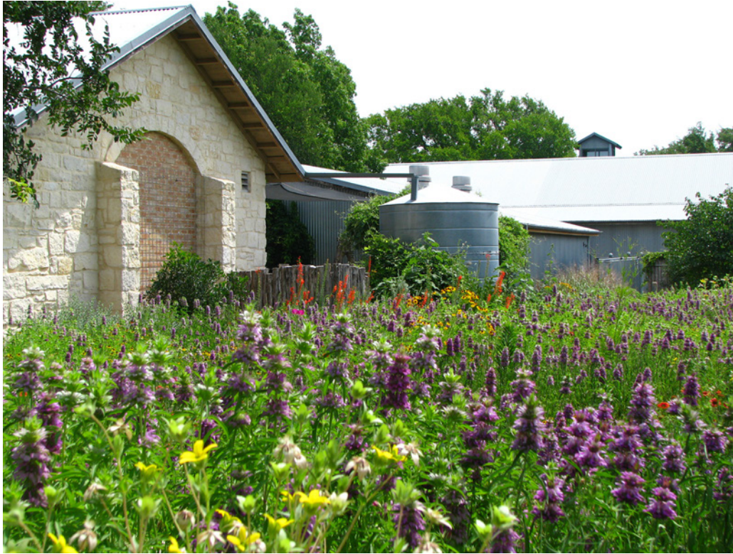
Figure 12. Lady Bird Johnson Wildflower Center: Sustainable Design. The Wildflower Center architecture is derived of the vernacular of the area and uses locally mined stone and adobe. Regular features of the Center are cisterns capturing rainwater from the heavy infrequent rains. (A. Hendrie)
