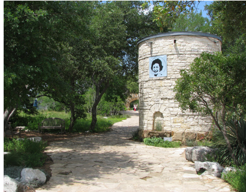
Figure 15. Lady Bird Johnson Wildflower Center: Entry Feature. The entry feature to the Wildflower Center is a large stone cistern connected to an aerial aqueduct. (A. Hendrie)
