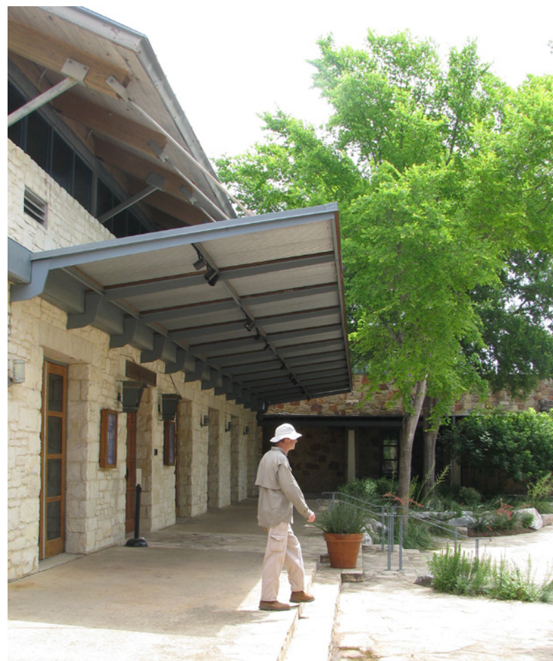
Figure 13. Lady Bird Johnson Wildflower Center: Architecture. Large overhangs made of tin provide needed shade and harken to the ranching barns of the area. (A. Hendrie)
