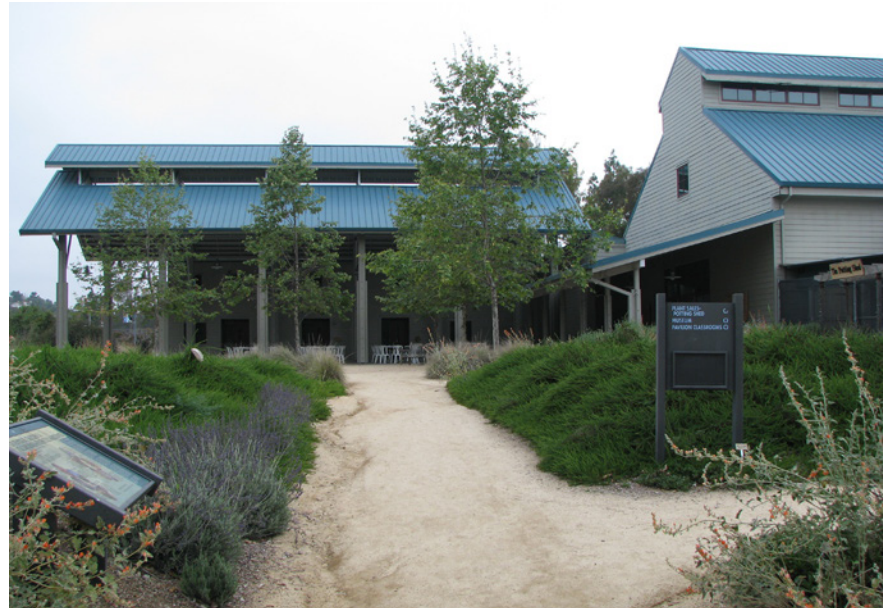
Figure 7. Fullerton Arboretum: Path Erosion. The only pedestrian path that leads to the pavilion space with the classrooms, museum, and nursery shows signs of erosion from irrigation and rain events. This decomposed granite path is not an ideal choice for this high use path. (A. Hendrie)
