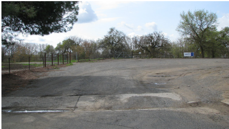
Figure 32. Equestrian Center Entrance. Sediment from the gravel driveway is carried by vehicles into the street. This is further enhanced after rain events. (A. Hendrie)
