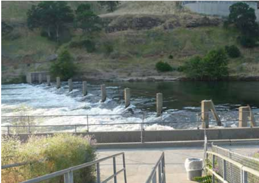
Fig. 6: Nimbus Fish Hatchery Weir
