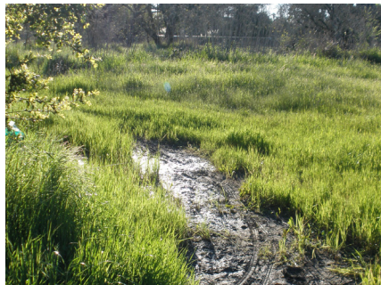
erosion trails & saturated soil near buried creek
