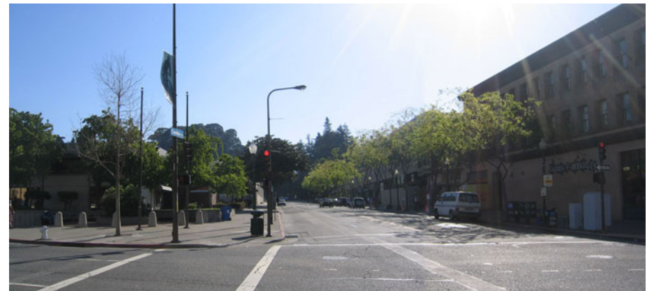
i.5 - Image of current Center Street condition looking East
