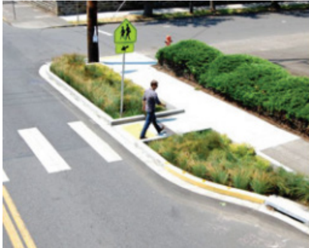
Image 2.9: Sidewalk Curb Bulbout (source: Perry, 2009)
