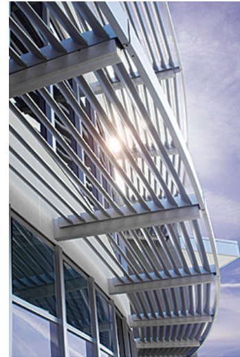
Image 2.5: External Window Shades (source: facilities.net)
