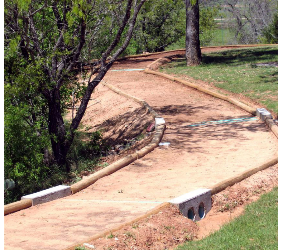
Figure 5.18: Decomposed Granite Path HAT -Handicapped Accessible Trail
