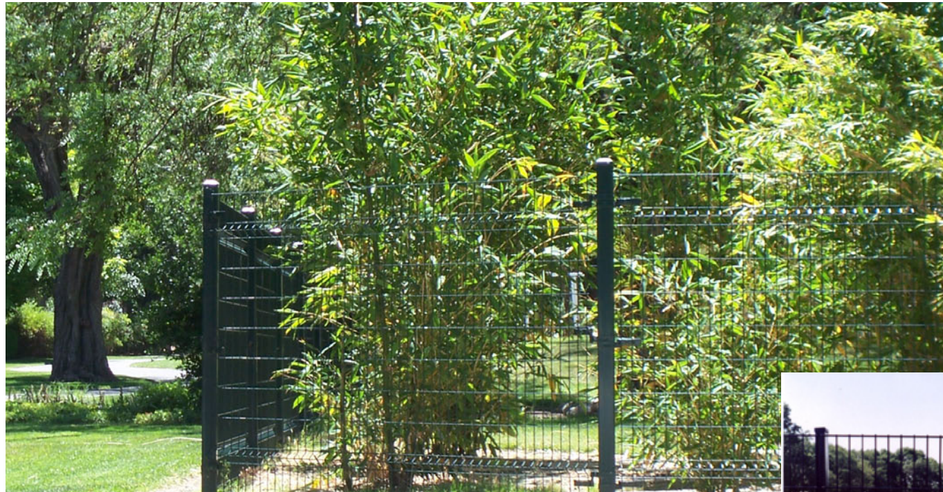
Figure 5.12: Wire fence example, UC Davis
