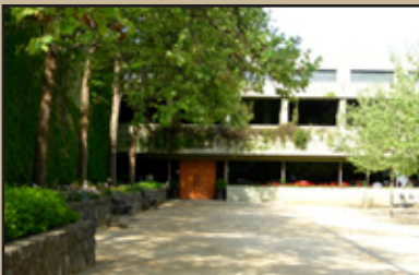
Building Architecture & Main Entrance
