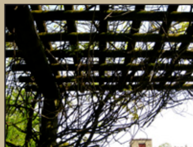
Trellis Shade Structure
