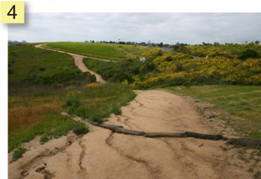
decomposed granite erosion Figure 3.5.
