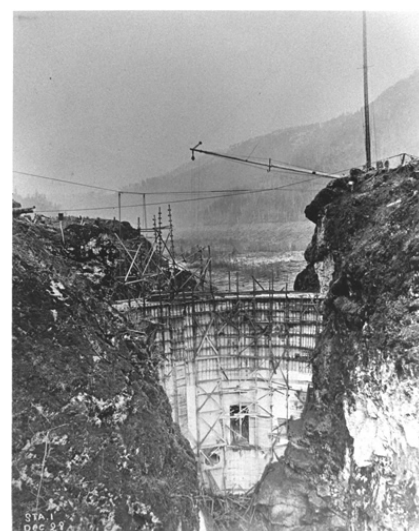
Figure 1.1: Elwha Dam under construction Paul. 2013.
