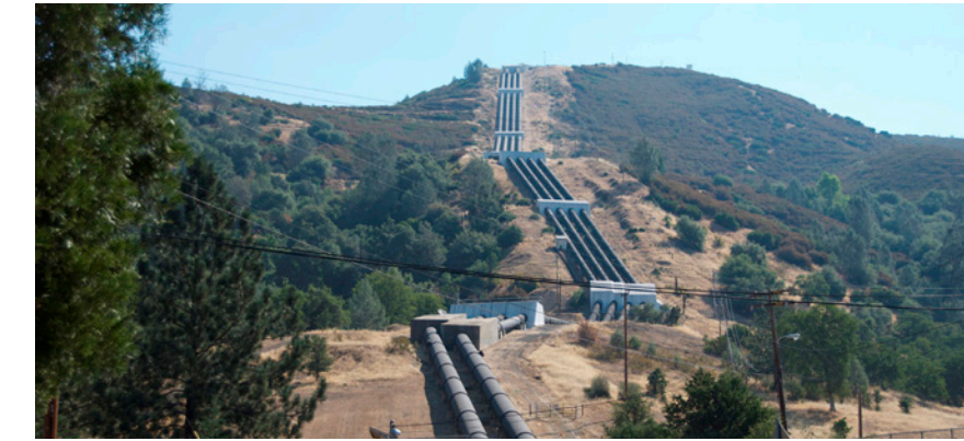
Figure 2.5: The Hetch Hetchy Aqueduct. Stretching over 167-mile. This gravity-driven network of pipes delivers 31,900,000 cubic feet of water daily to S.F. Aquaforia, 2008
