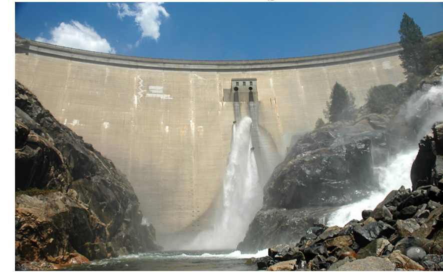
Figure 2.6: The O'Shaughnessy Dam. At 312-foot-high, millions of gallons of pristine mountain water are retained for the citizens of the Bay Area. Aquaforia. 2008
