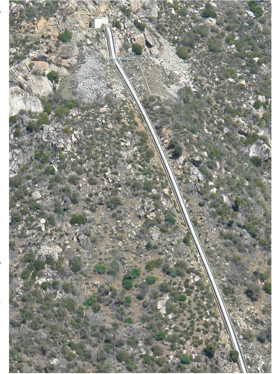
Figure 5.1: Gravity-propelled Aqueduct. The Hetch Hetchy Aqueduct pays homage to man’s innovation and engineering, but at the price of ruining a beautiful mountain side. This is a part of the aqueduct coming from Cherry Lake. Carson Cooper, March 24, 2013.
