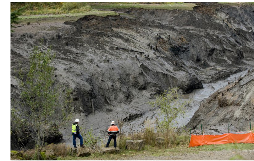
Figure 4.3: A River Cuts Through It. Much of the channel restoration was given to natural processes: using the force of the river, gravity, and properties of water allowed the river to make its own channel. www.columbian.com, 2013.
