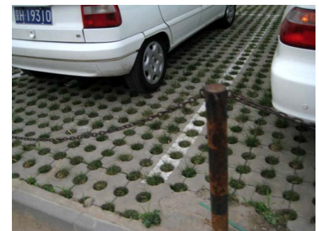
5.4 permeable parking lot pavers
