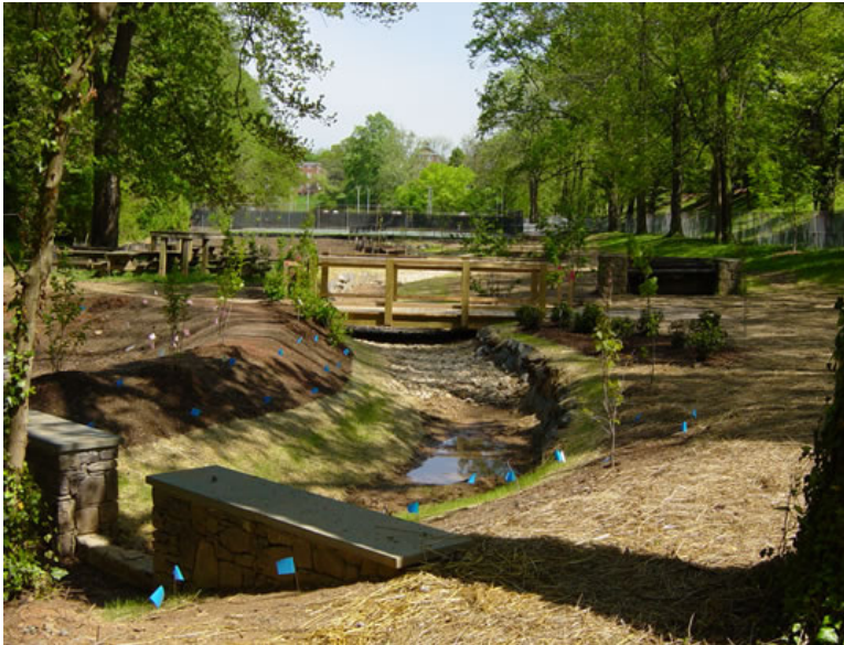
Figure 3.0: Meadow Creek Day-Lighting project
