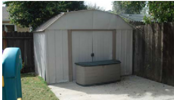
Fig. 6.13: The Existing Storage area. (Arrow G)
