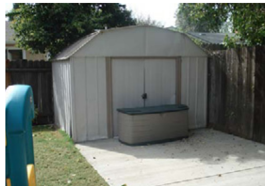
Fig. 5.3: Looking from the concrete pathway to the storage area.
