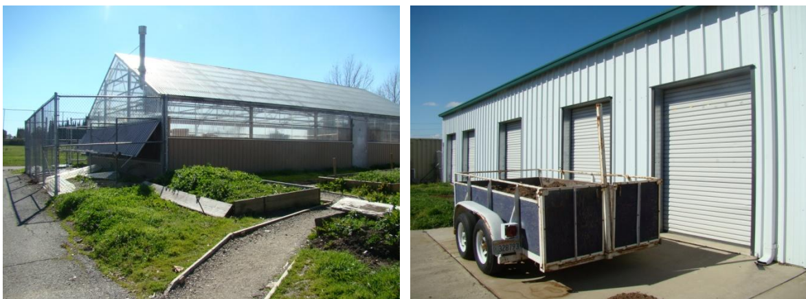
Figure 5.4 7 5.5: View from the main entrance & view of the barn
