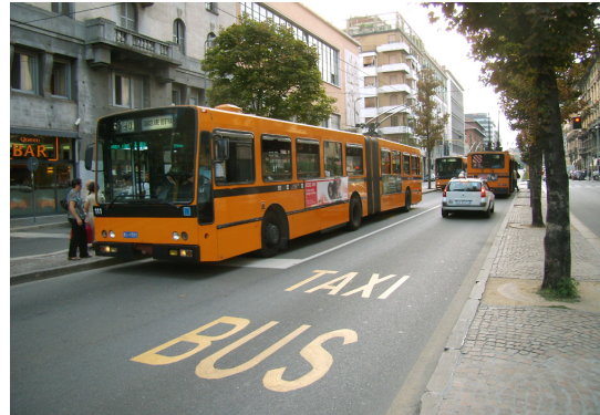
Figure 1.7 Converted Bus-Only Lane The next step below designation is conversion. When speed is only crucial during specific times of the day like rush hour, curbside lanes can be converted for only part of the day (Fig. 1.7). This requires faith on the side of other vehicles and possible enforcement for assurances but is capable of providing higher bus speeds at very low capital costs.
