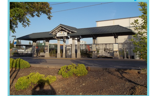
Figure 2.14 SRT Gold Line (LRT) - Sunrise Station
