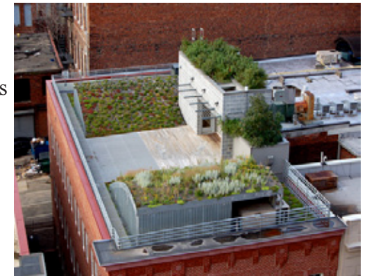
FIGURE 18 ASLA ROOFTOP AERIAL VIEW
