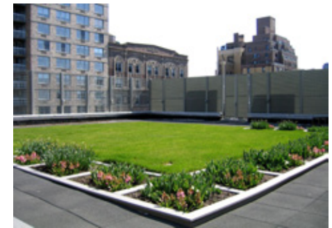
FIGURE 7 SEMI-INTENSIVE ROOF ABOVE CALHOUN BUILDING
