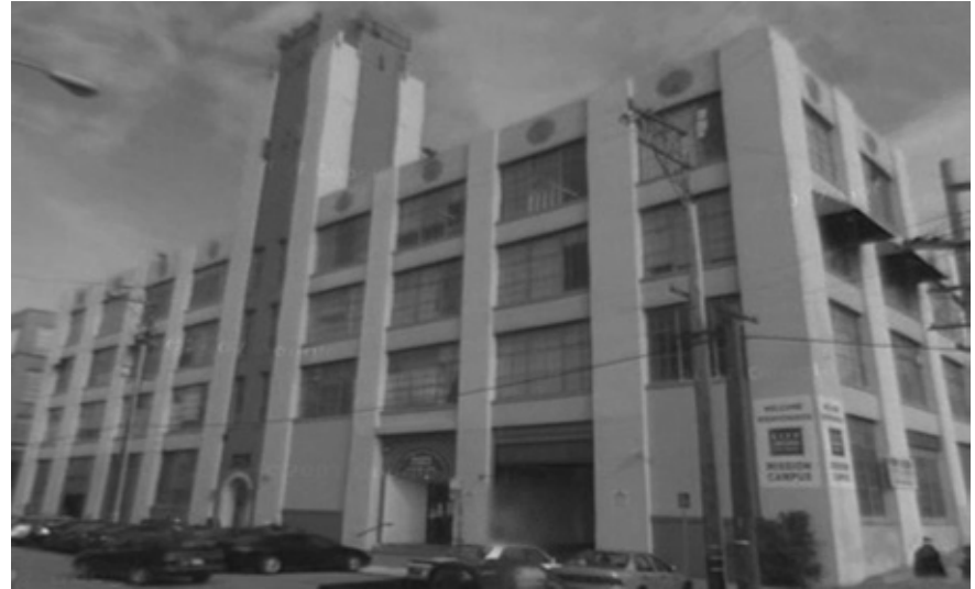
FIGURE 28 ALABAMA STREET BUILDING
