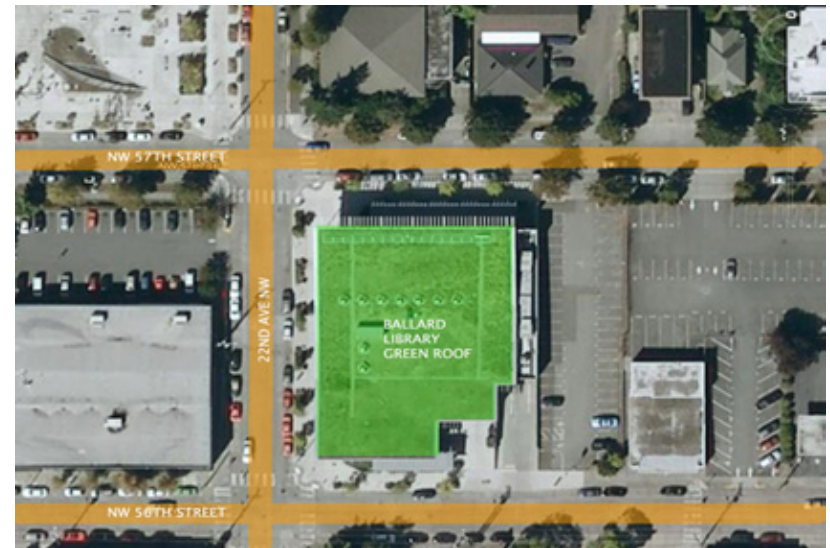
FIGURE 23 SEATTLE BALLARD LIBRARY EXTENSIVE ROOF
