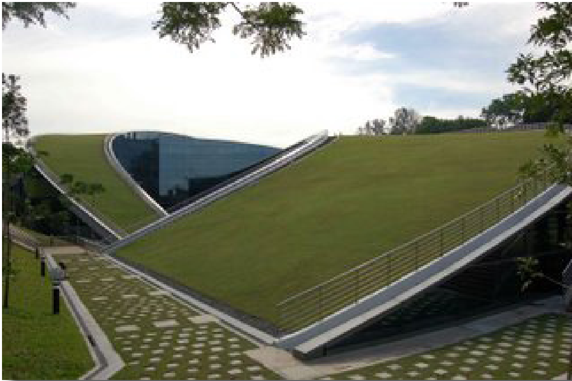
The School of Art and Design in Singapore is an example of a simple-intensive green roof
