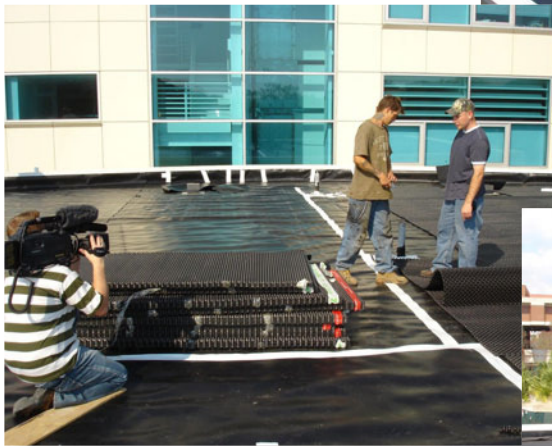
Root Barrier and Drainage Layer
