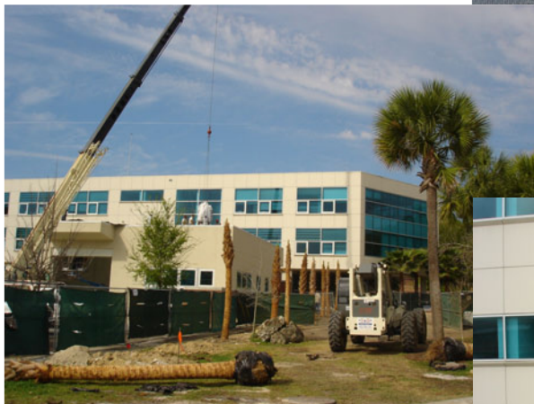
Materials Hoisted with Crane
