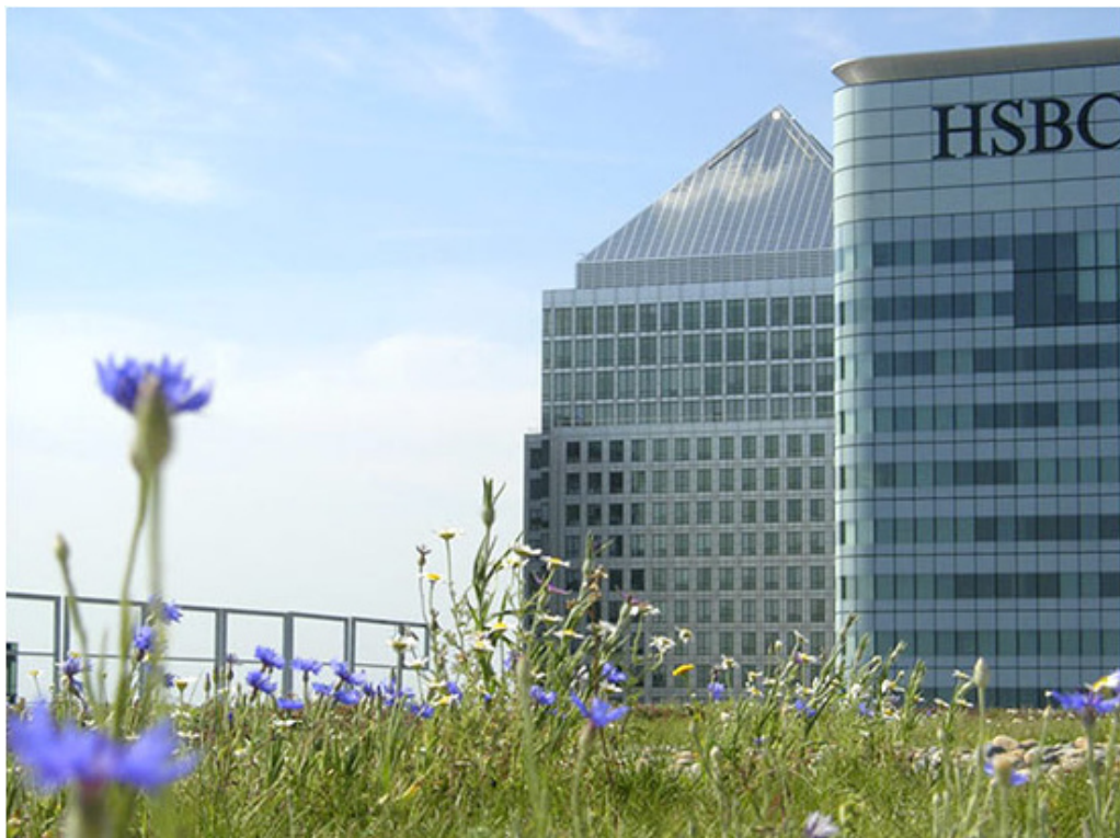
A green roof planted with wildflower and grassland seeds, Barclays Headquarters, London
