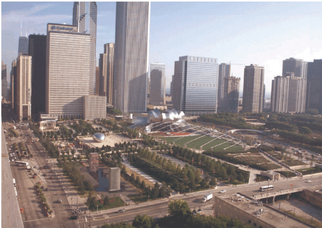
Millennium Park in Chicago is a 24 acre green roof that sits over a parking garage.
