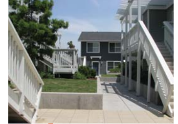
upper story corridor
