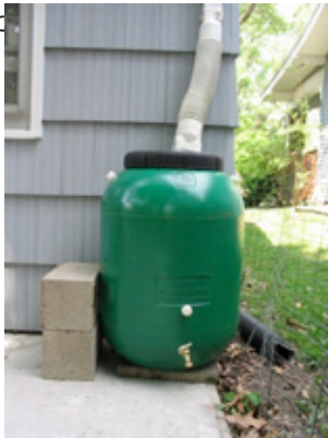
3.4 - Rainwater barrel attached to roof storm drain
