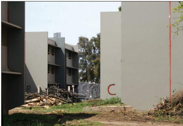
Figure 9: Photograph of Site Demolition
