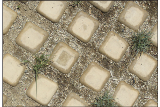
Figure 22: Another Example of Permeable Pavement
