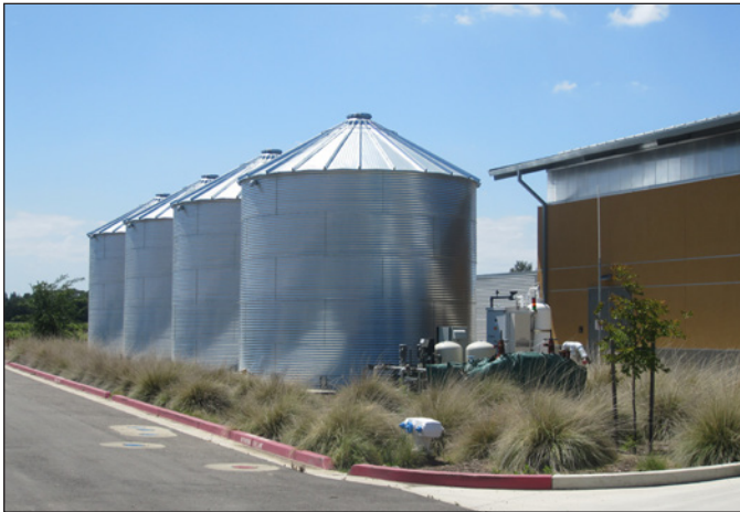
Figure 34: Rainwater Harvesting Collection System
