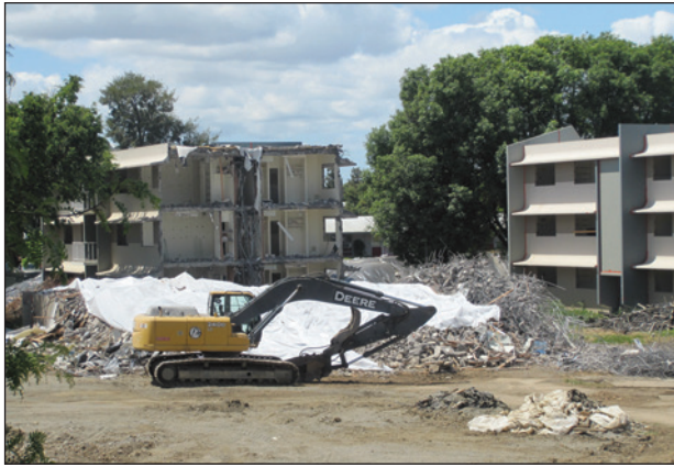
Figure 8: Photograph of Site Demolition
