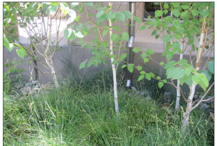
Figure 23: Bioswales Designed to Capture Stormwater Runoff From Pavement and Roofs
