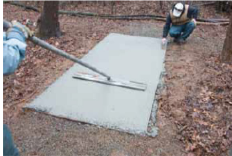
Float the concrete to force rocks down. It will help with texturing.
