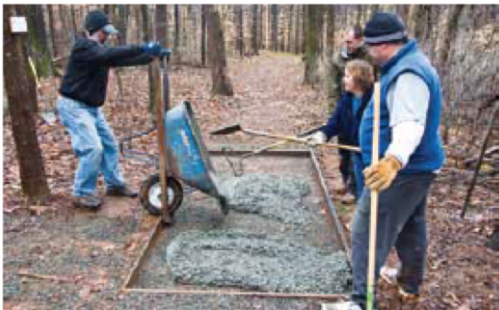
Use wheelbarrows to transport concrete to tees in remote areas.
