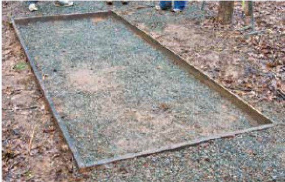
Frame is ready for concrete.
