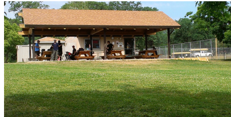
Figure 16. Resting area at Shady Oaks course in Orangevale, CA
