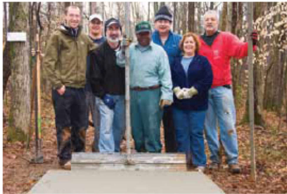
A prepared gang of workers makes tee construction easy.
