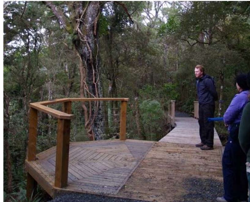
Figure 5.13: The viewing platform might look something like this one, but instead of mesh in between the wooden poles, I recommend using wooden panels. Source: http://sciblogs.co.nz/science-life/2009/10/29/orokonui-ecosanctuary-to-open/
