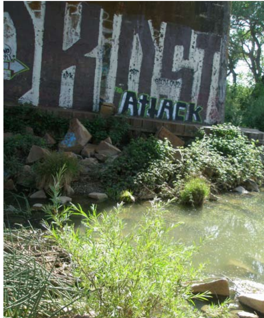
Figure 4.11: Graffiti under the railroad bridge.
