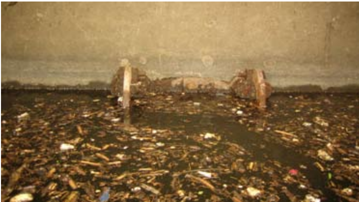
Top: Figure 4.7: Outflow pipe into Putah Creek
