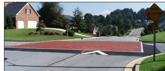
Figure 1.19 Raised intersection
