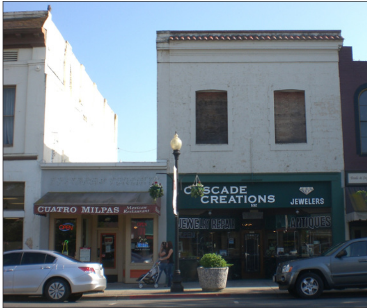
Figure 3.18 Wells Fargo Express Office building 2010
