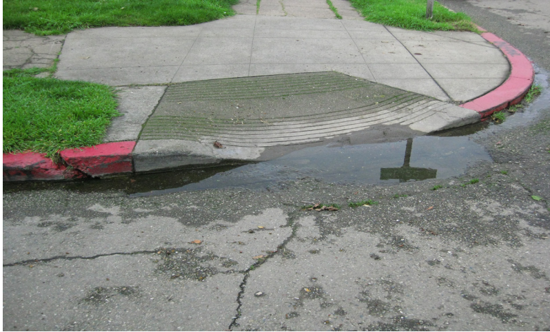
These photographs show the sorry state of drainage on Park Boulevard. fig. 6: a flooded access ramp, fig. 7: a previously flooded access ramp, now covered with debris. fig. 8 a catch basin covered with debris.
