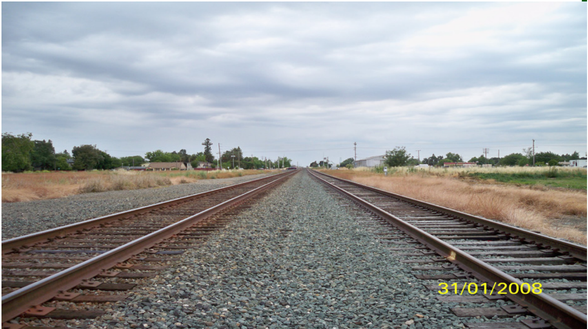
Fig. 5.1 Existing Rail Road Tracks
