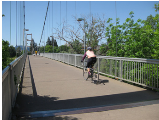
Figure 18. Guy West Footbridge
