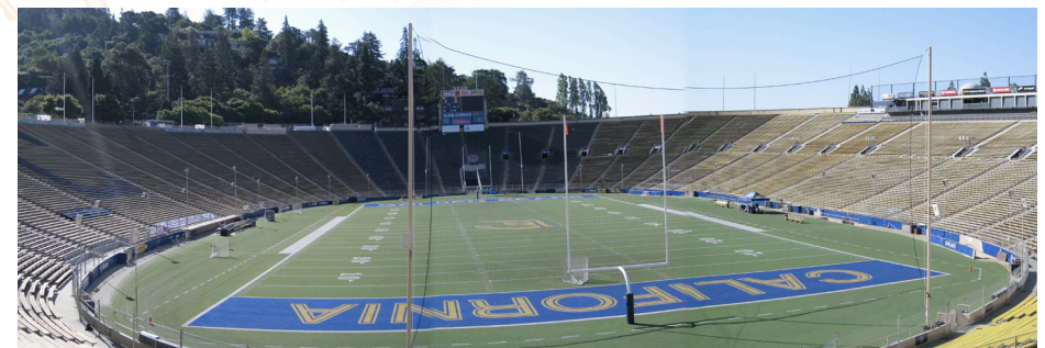
Photos: A panoramic view of Memorial Stadium (below). Bear claws walk across the walls creating the feeling of being in a bear’s lair (left).
