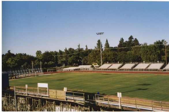
Image 1.9: Although historic, Toomey Field has slowly deteriorated over time.
