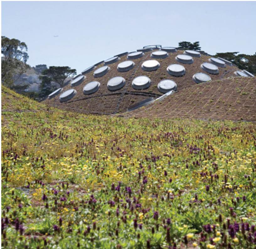
7.1. The California Academy of Sciences green roof under construction
