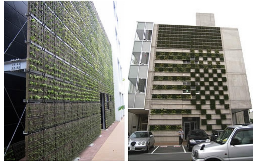
3.3. A living wall in Japan with a strong gridded feel (The Greenroof Project Database, 2006)
