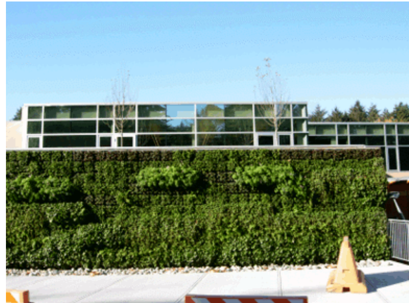
6.1. Aquaquest's living wall (The Greenroof Project Database, 2006)
