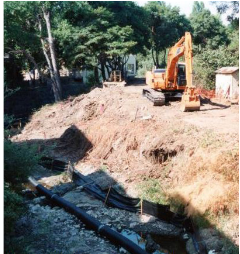
Figure 14: Construction on 1999 San Luis Obispo Creek habitat enhancement project
