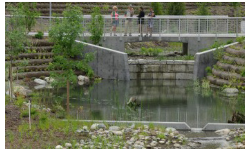
Figure 17: Wetland terraces clean storm water
