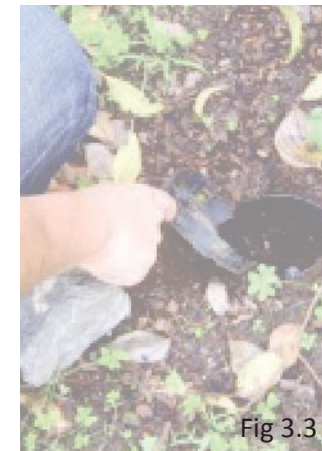
Below: Various terminals around his backyard for greywater subsurface irrigation
