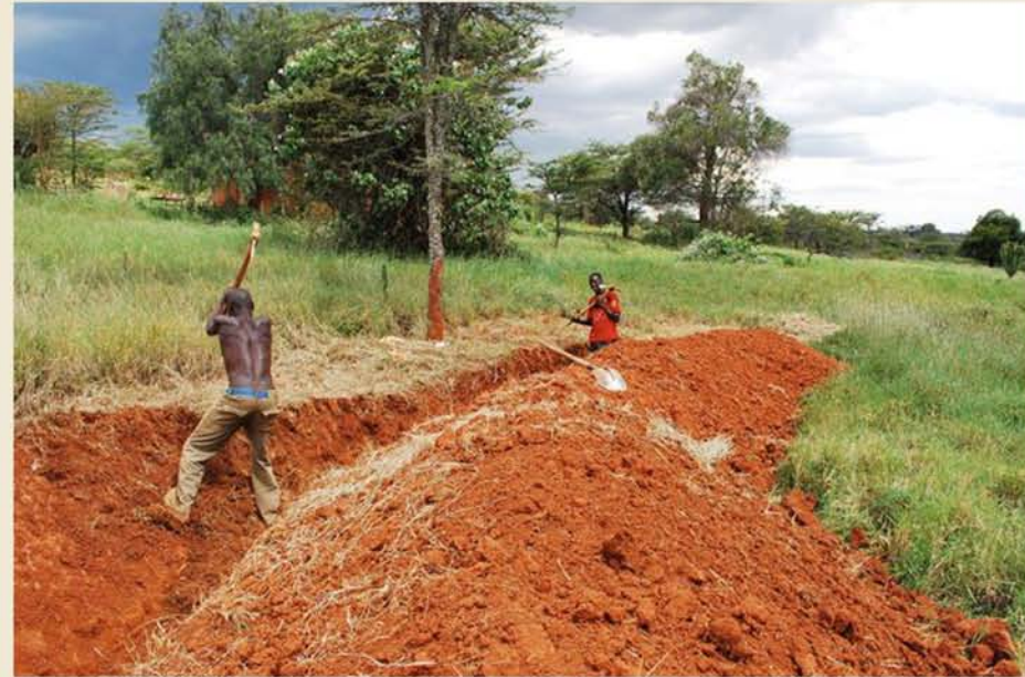
Figure 6.1 Digging Swales
