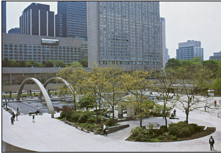
Fig. 4.2: This entire urban plaza, complete with mature trees and institutional art, is actually a large green roof designed to carry heavy loads.
