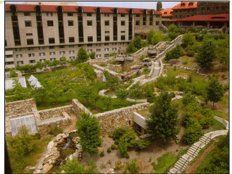
Fig. 4.1: This entire landscape, complete with trees, walls and walkways is actually an intensive green roof. The design allowed the Grove Park Inn Resort and Spa in Asheville, NC to develop the center of its U-shaped complex, increase its usable space and draw in the area's natural beauty.
