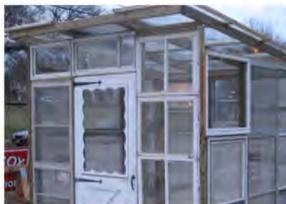
Tricycle Gardens HQ - reused window greenhouse. (Tricycle Gardens, 2011)
