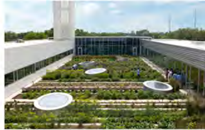
Rooftop Haven for Urban Farming (Levenston, 2010)
