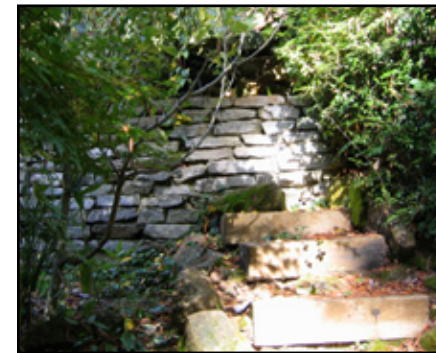
Fig. 7.9 Dry-stacked stone wall
