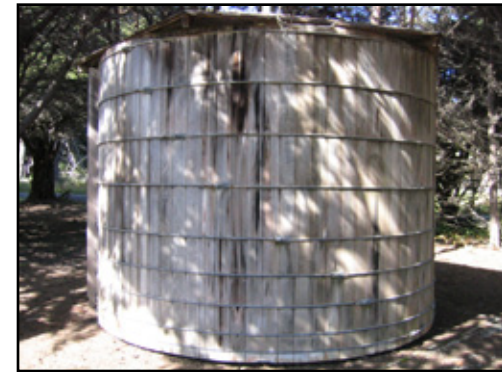
Fig. 7.12a Water storage cistern made in Healdsburg, CA
