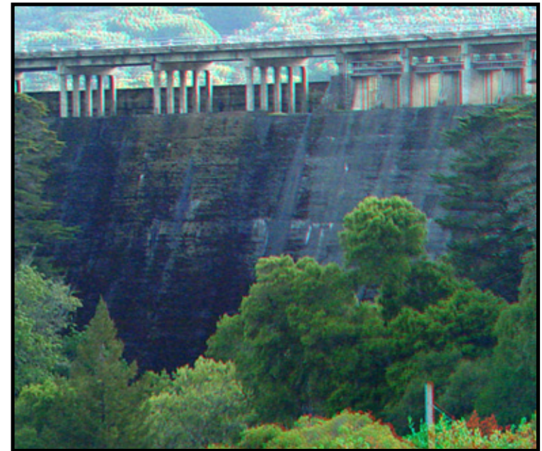
Fig. 1.3 and 1.4 Crystal Springs Reservoir and Dam
