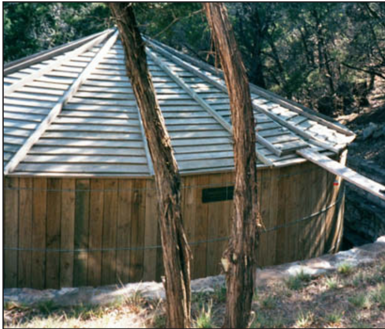
Fig. 7.11 25,000-gallon Timbertank in Central Texas - showing the rustic aesthetic appeal of wooden tanks.
