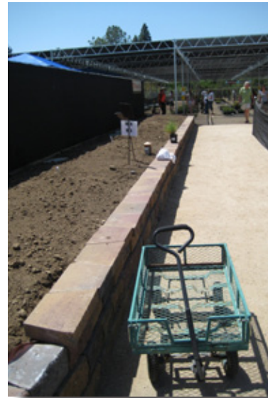
Photo 5 - Pollinator Demonstration Bed with built seat walls, rounded corners and soil fill
