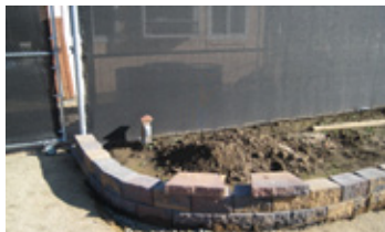
Photo 7 - Partially built demo bed wall
