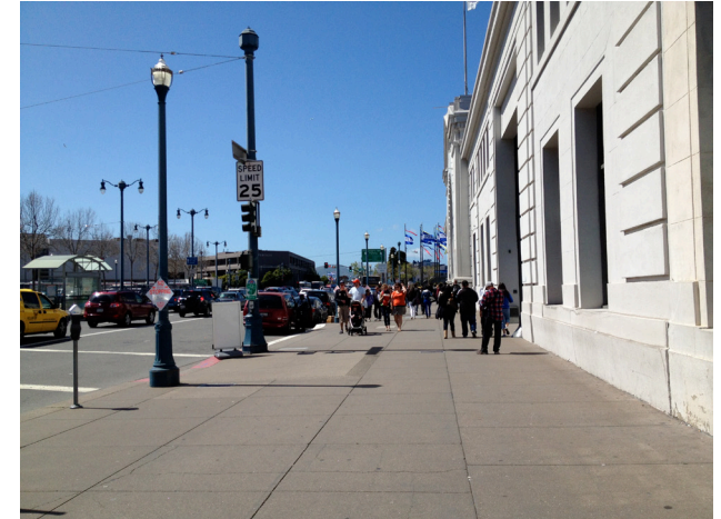
Fig 7.8: Mass of concrete sidewalks and piers
