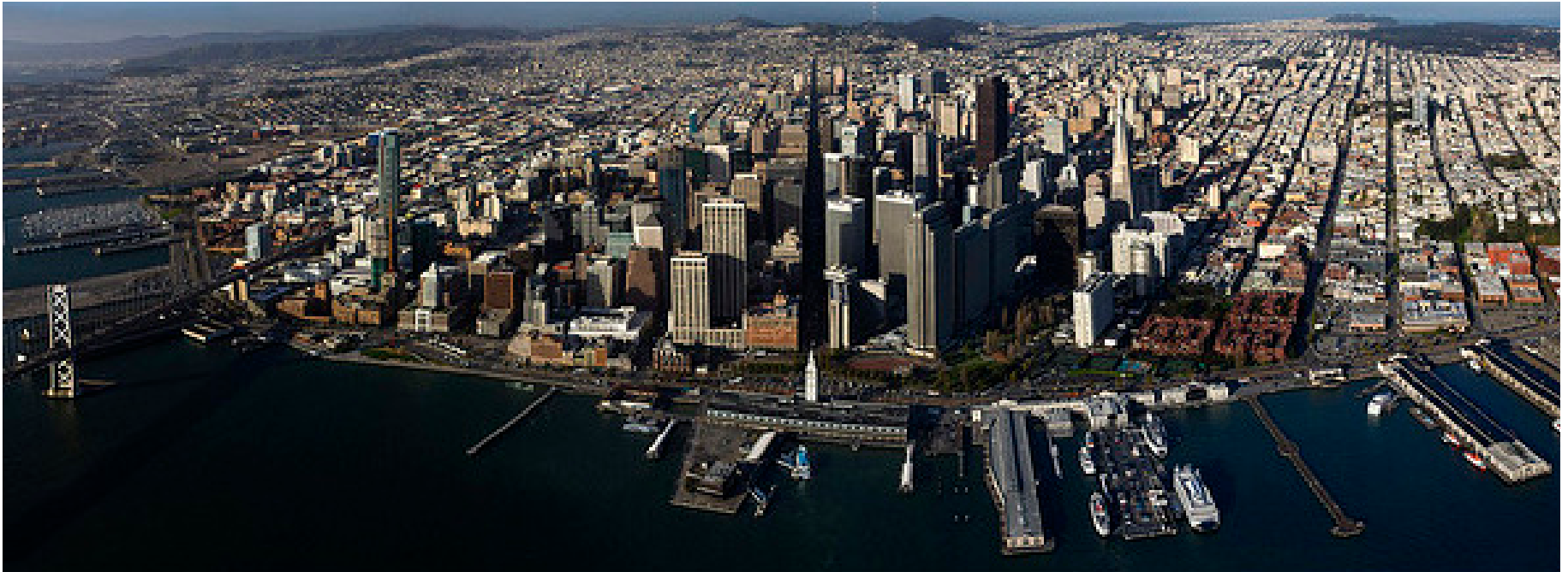
Fig 7.24: Span of The Embarcadero
