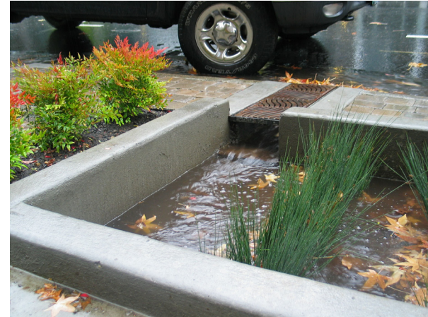
Fig 6.8: Stormwater Planter Curb Detail
