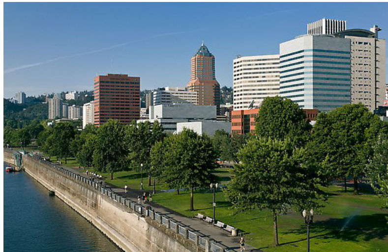
Fig 6.4: Seawall at Tom McCall
