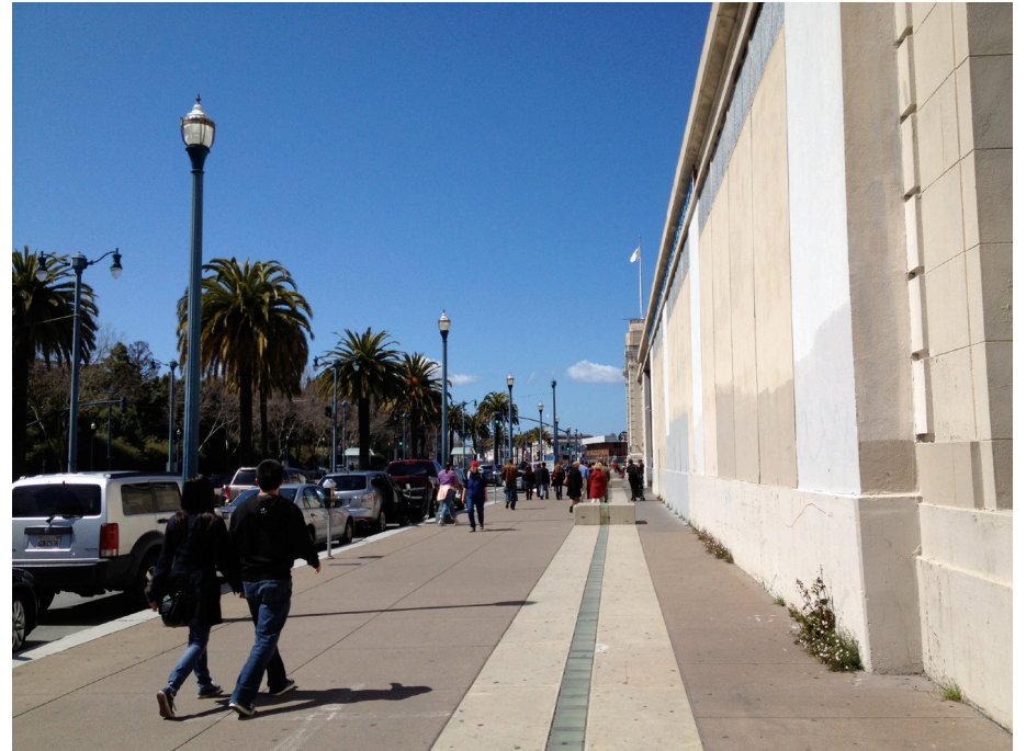
Fig 3.2: Concrete Piers of The Embarcadero
