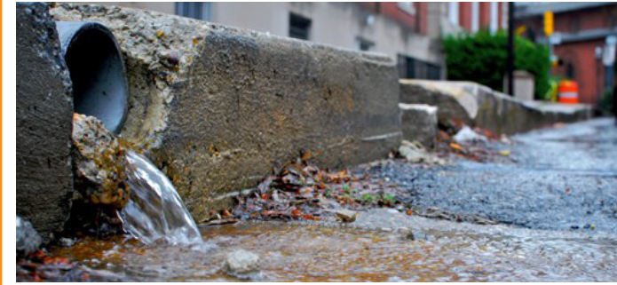
Fig. 1.12 Stormwater flowing onto the street.
