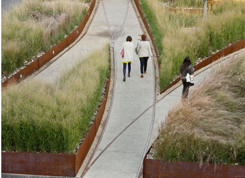
FIG. 3.10 Aerial of rails incorporated into concrete pathways
