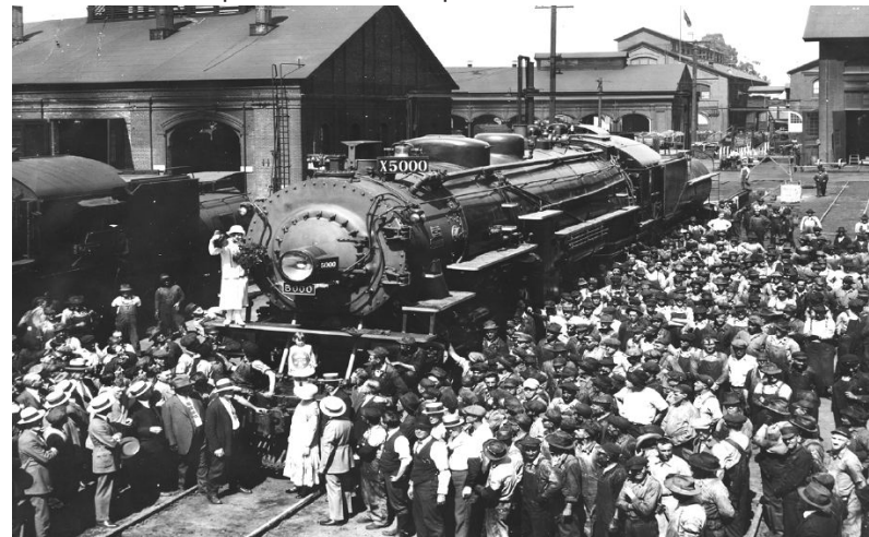
FIG. 2.1 Southern pacific railroads shops
