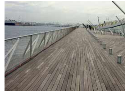
3.2 - Boardwalk on Ferry Terminal
